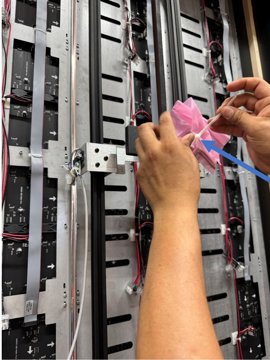
Cut this tie wrap to free car and use hardware in plastic bag to secure backbox to main cabinet.
